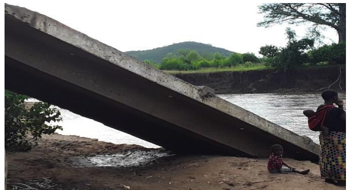
Bridges destroyed by the heavy rains and floods
